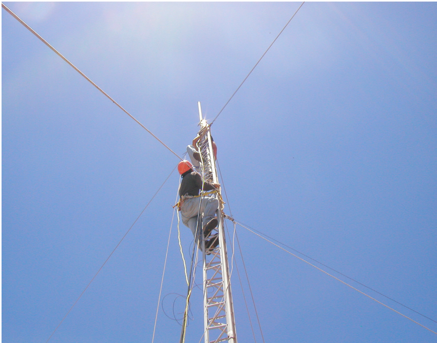
Figure 7.2: A climbable guyed tower.
