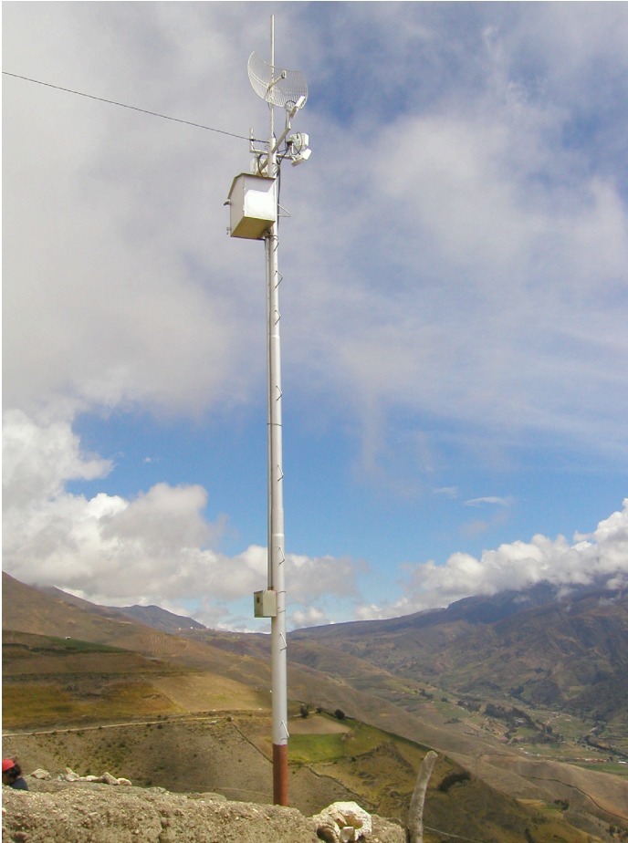
Figure 7.3: A simple self-supporting tower.
